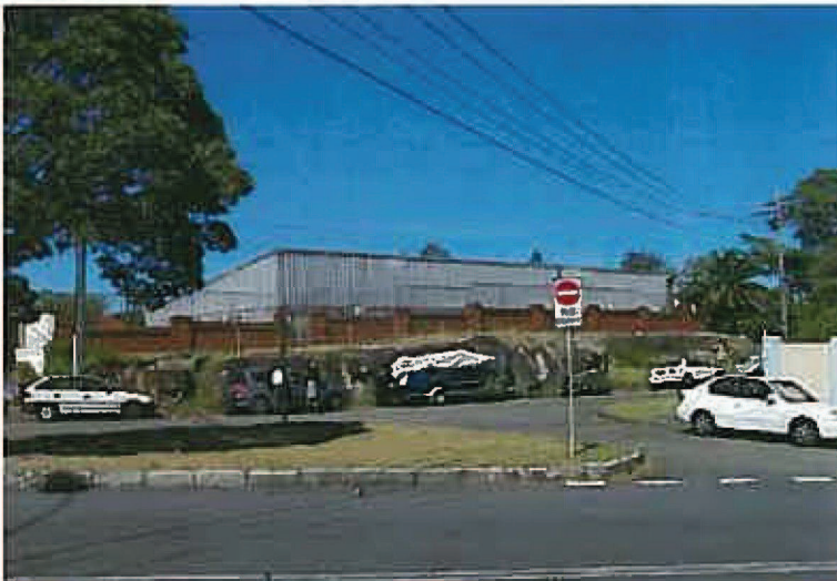
Figure 4.8 View of the redundant Manly Reservoir, looking from Hilltop Crescent. Note that the principal fabric visible from the streetscape is the 1960s metal clad roof structure.
