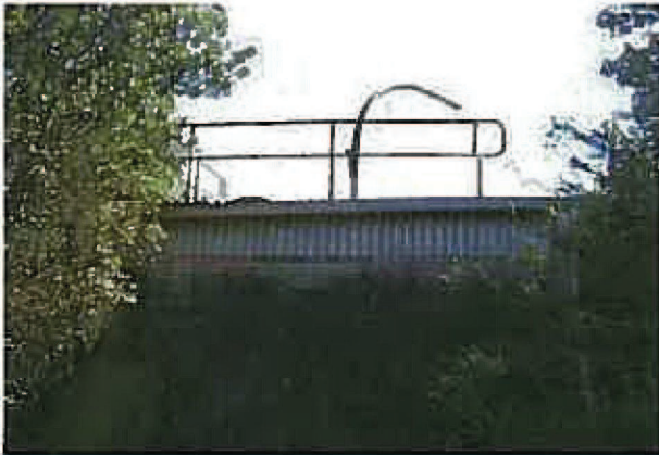
Figure 4.18 South west corner of the reservoir
