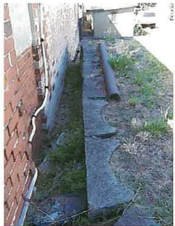
Figure 4.27 Detail showing position of former pumping equipment
