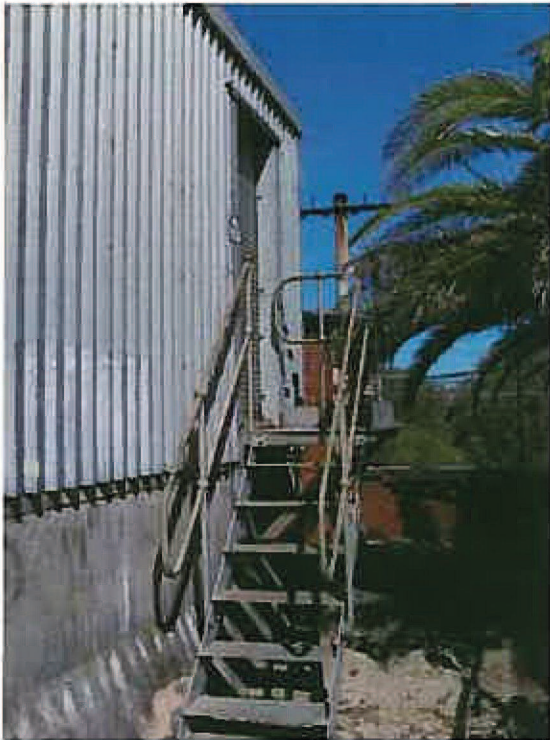
Figure 4.24 Postwar access ladder on the side of the reservoir
