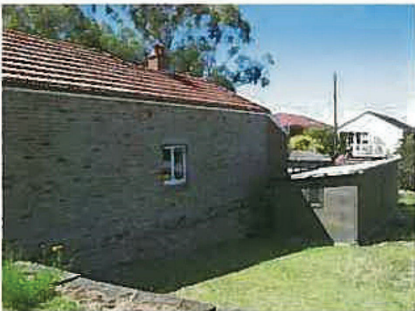
Figure 4.20 Residential dwelling adjacent to (east of) the reservoir site and storage/equipment shed within the site
