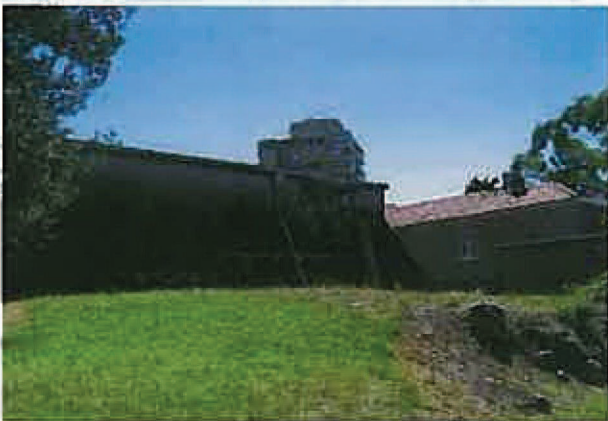
Figure 4.12 Site view of the Manly Reservoir structure
