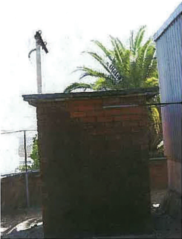
Figure 4.23 Reservoir detail, likely to have been carried out at the same time the reservoir was enclosed (1960s)
