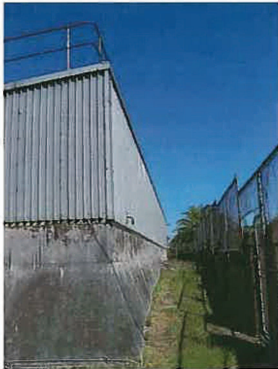
Figure 4.26 View along the side of the reservoir
