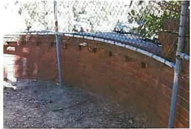
Figure 4.17 Detail showing part of the curved 1920s fence
