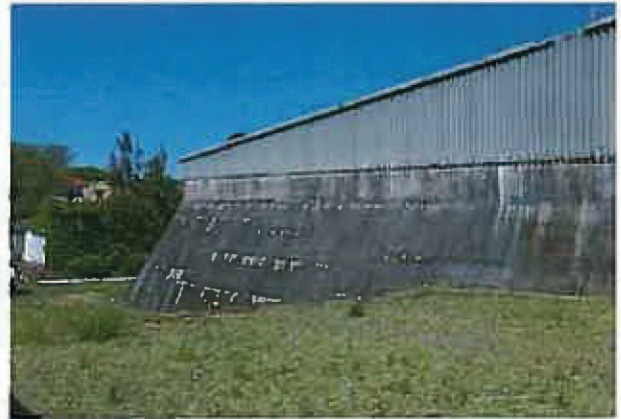
Figure 4.19 View from terrace showing the south east corner of the reservoir
