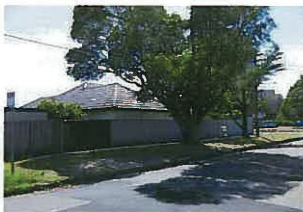
Figure 4.3 Single storey residential development at the corner of Fairlight Street and Hilltop Crescent, directly opposite the site
