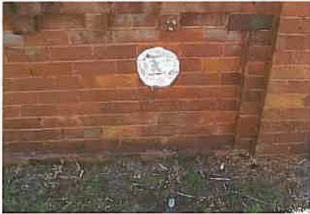
Figure 4.16 Detail showing part of the interwar-era brick fence
