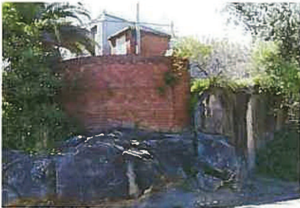
Figure 4.10 Corner of the subject site, at the intersection of Fairlight Street and Ashley Parade
