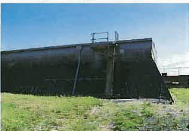
Figure 4.14 View of the rock and concrete reservoir structure showing access ladder and drainage
